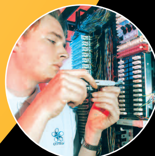
Termination Techniques and Commissioning
